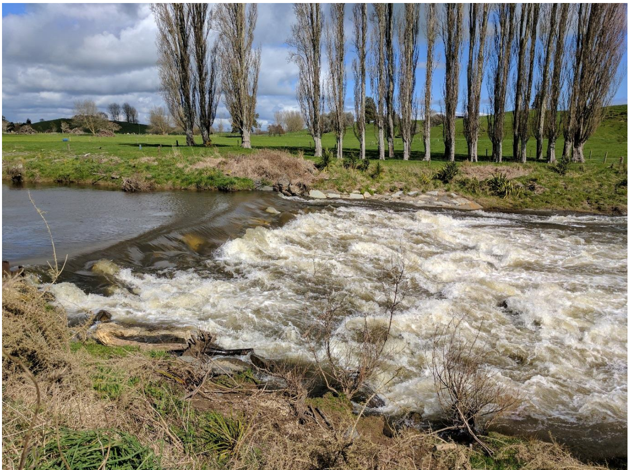
An example of a rock-ramp style weir that also has a fish pass along the true left bank.
